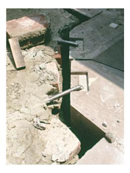
FIGURE 28. The 1 inch (2.5 cm) gap established between the bick structure and the new stone (actually coloured concrete) decorative elements. Sensors were placed in this gap and at other places in three sections through the building.
