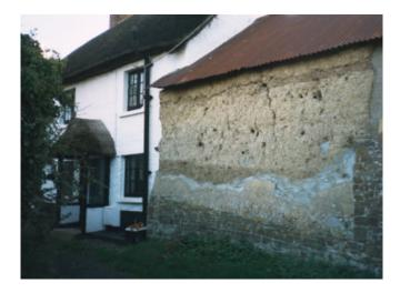
FIGURE 32. A slowly disintegrating earth building in central Devon. The tin roof and the stone base to the wall ensure surprising durability even against driving rain, frequent fog and an unheated interior.
