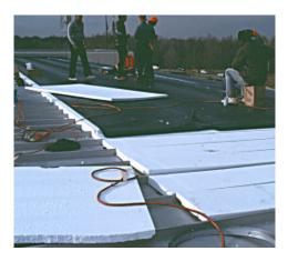
FIGURE 21. Polystyrene insulation being put on the roof of the street shown in the previous figure.
