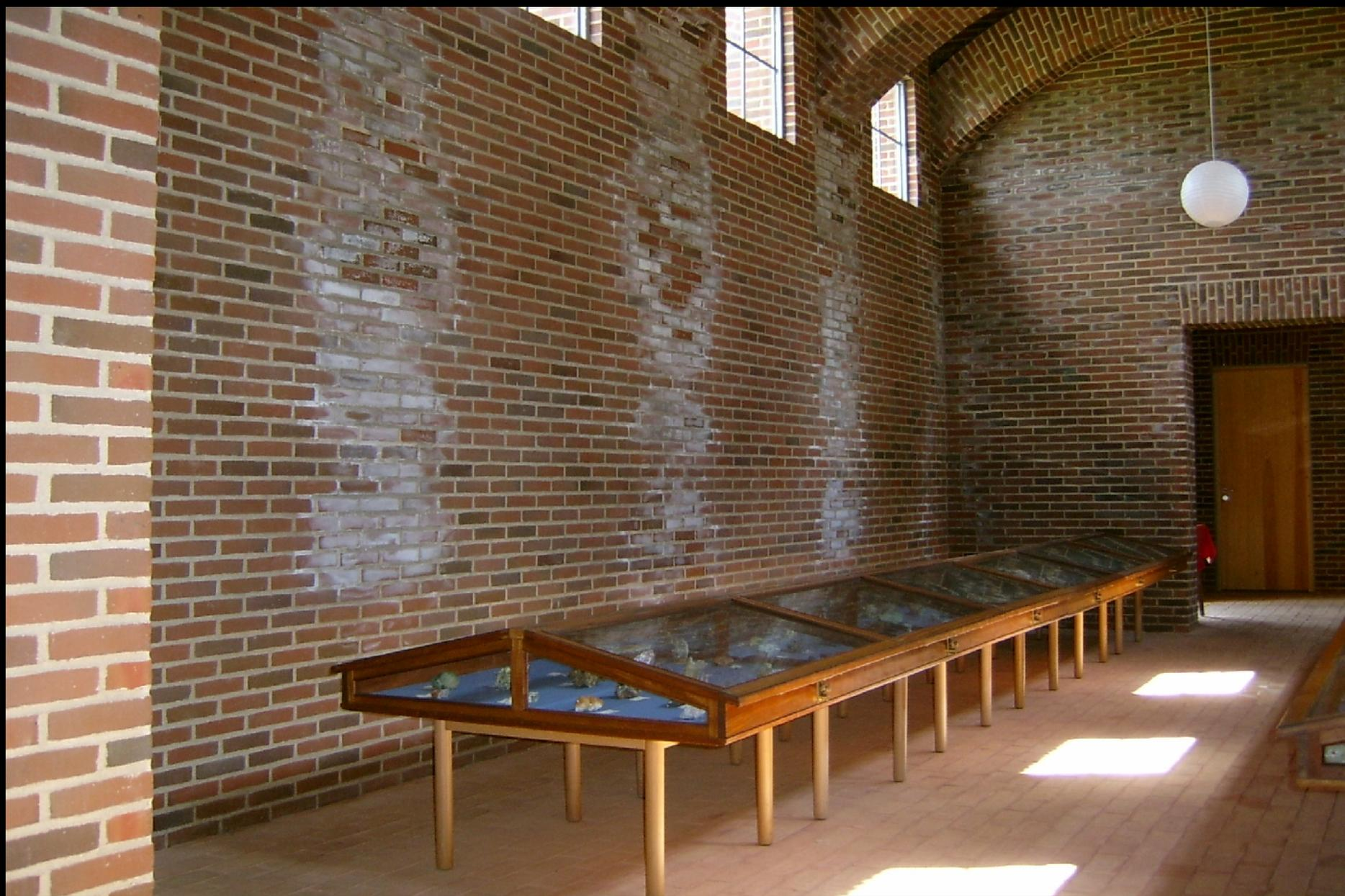
The white salt efflorescence shows where rainwater is leaking through.
