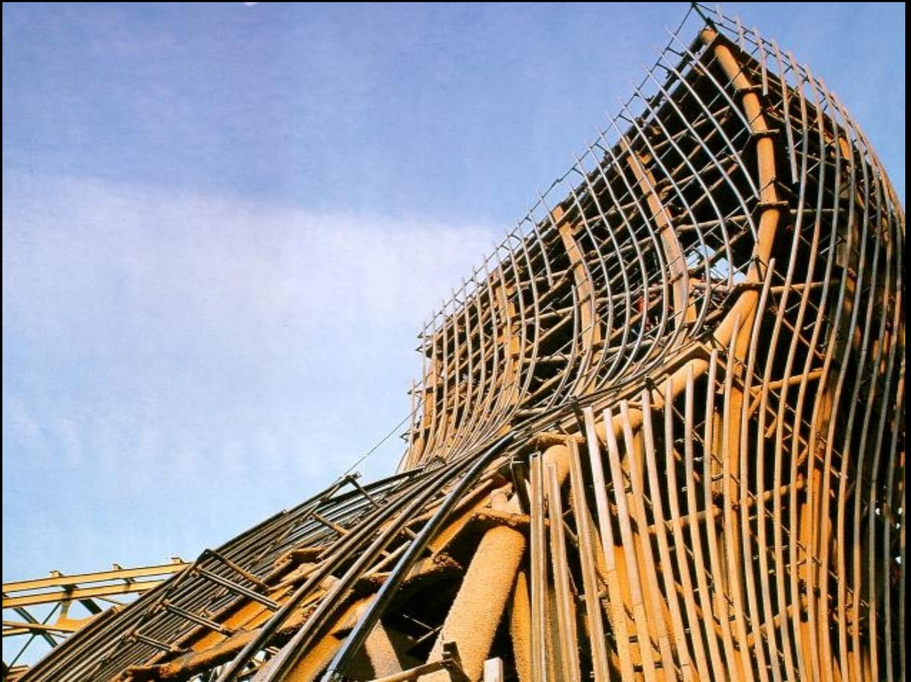
The steel framework forming the curved shapes of the building
