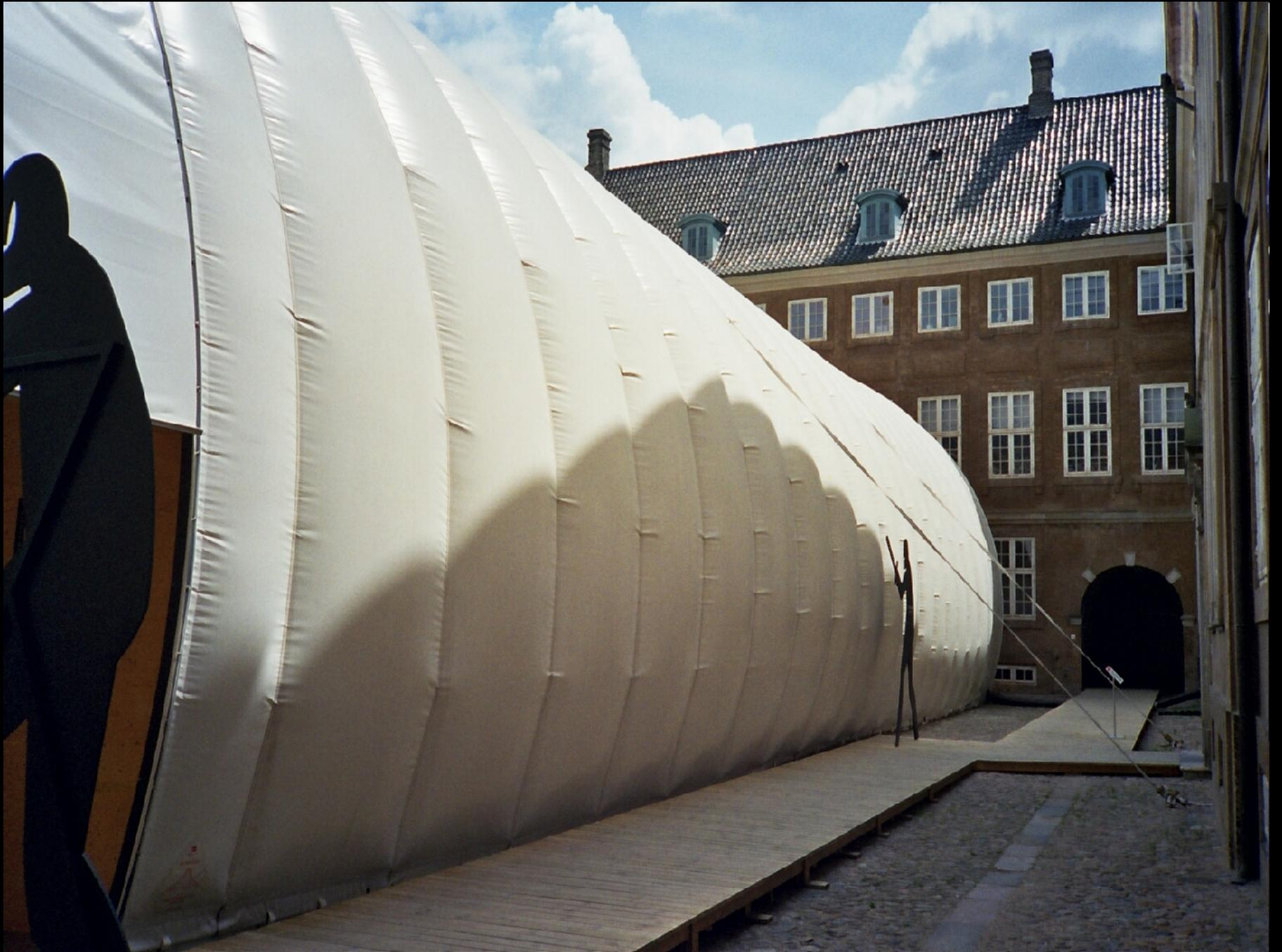
The pressurized structure was leaking air though the doors and floor
