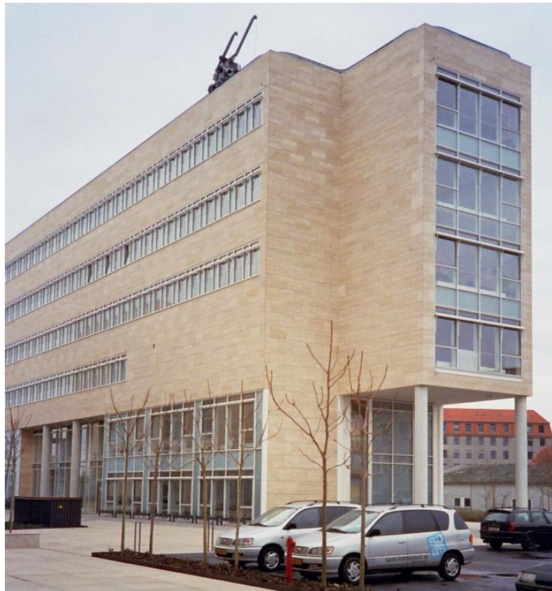
Figure 1: The building in Copenhagen University which houses the Arnamagnæan Institute. The archive is the room behind the windowless portion of the long facade.
