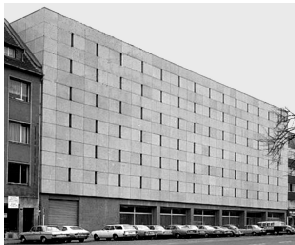
Figure 3: The City Archive in Cologne (1971) was designed with thick outer walls for thermal inertia. The interior was heated and ventilated to control the RH.
