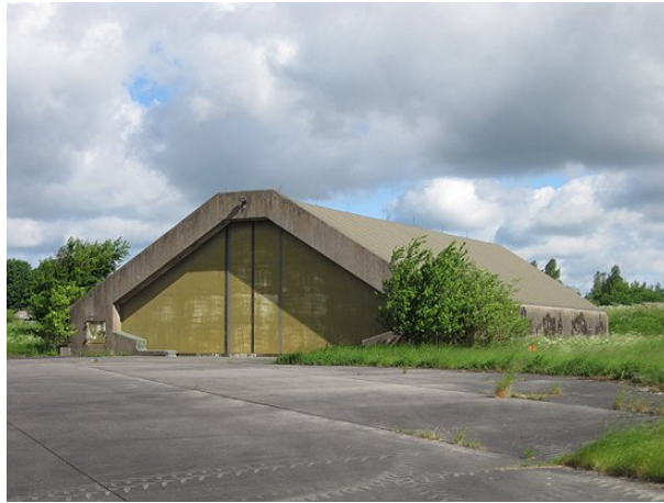
Figure 8: The solid concrete shelter for fighter airplanes at Værløse, Denmark, now used as a temporary store for a collection of historic furniture. The annual temperature variation is 0–25 °C and the RH is controlled to 50% by dehumidification.
