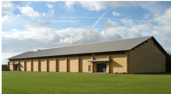
Figure 10: A well insulated museum store for a local museum collection in Ribe (2006). The annual temperature variation is 8 – 16 °C and the RH is controlled to 50% by dehumidification.
