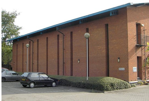
Figure 4: The Suffolk Record Office, Ipswich, UK (1990), had winter heating to 16 °C. The RH was stabilised by the humidity buffer capacity of the documents.
