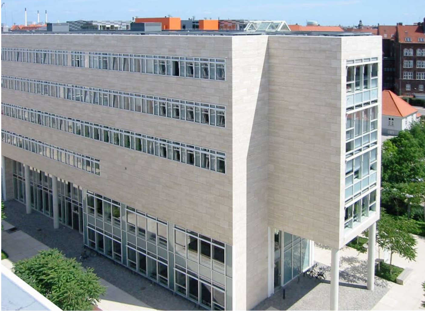
Figure 3. A building of Copenhagen University. The Arnamagnæan archive is behind the portion of wall without windows. It has no internal heating but gains heat from the core of the building, which is kept within the human comfort zone. Heat loss to the outside through thin insulation on the two exterior walls keeps the archive temperature about midway between indoor and outdoor temperatures. Photo: Morten Ryhl-Svendsen.
