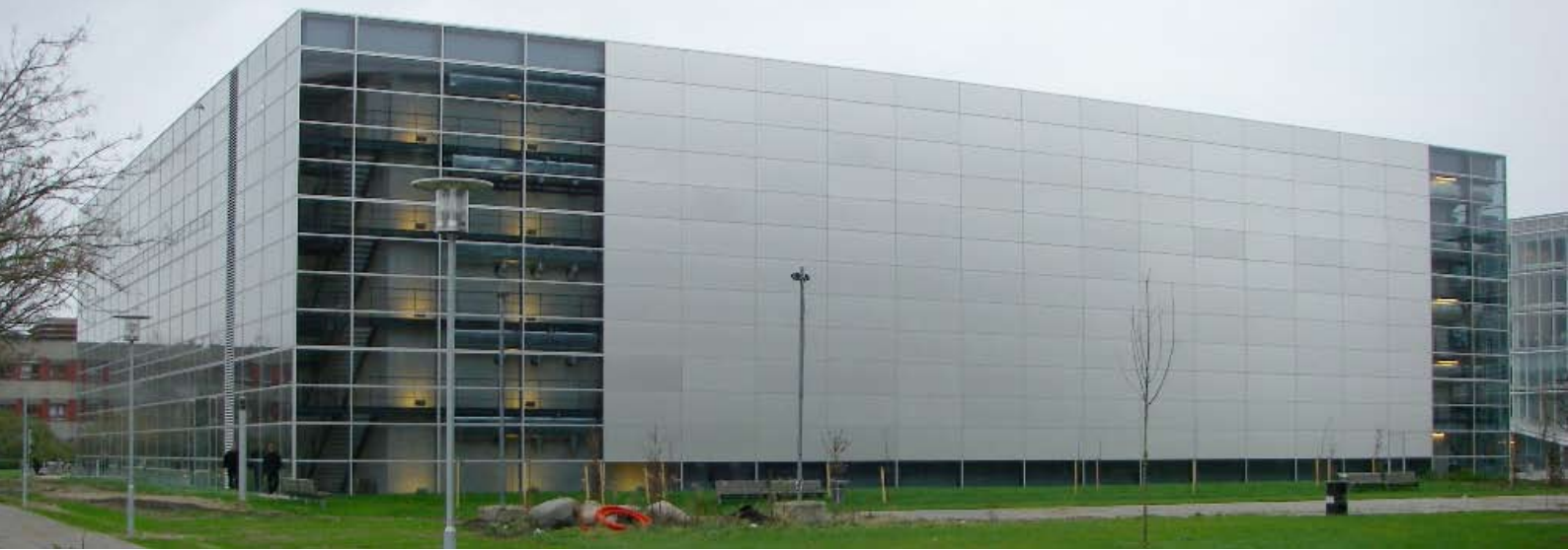
Figure 1. A storage building of the Royal Library in Copenhagen, about 6,000 m 2 , completed in 2000. It is permanently air-conditioned to a set point at 18°C and 50% RH. Photo: Lars Aasbjerg Jensen.
