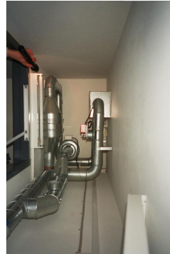
Figure 65: The minimalistic air conditioning equipment.
