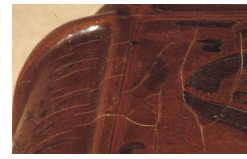
Figure 27: A close-up of the box of figure 26, showing cracking across the longitudinal direction of the wood support.
