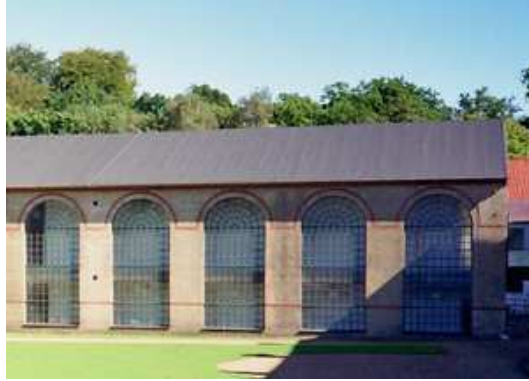
Figure 19: A museum store in Brede, north of Copenhagen. A new, thermally insulated, airtight and moisture buffering room has been built within an old machine hall, leaving a corridor between the old shell and the new room. Climate control is by heating and by pumping outside air into the room when the water vapour content is suitable.
