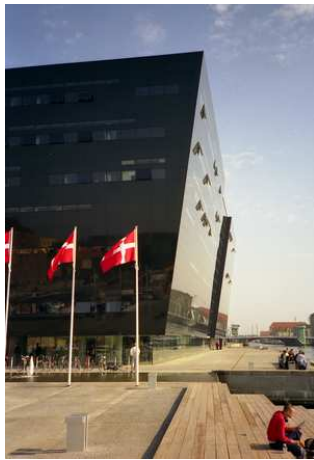
Figure 3: The Royal Library extension, Copenhagen, 1999. Designed by Schmidt, Hammer and Lassen.
