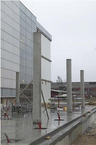
Figure 3. The building site with the original façade of block 1 and the additional constructions to support the new façade. (The Royal Library)
