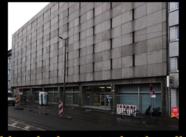
The building had massive brick walls filling a concrete frame. An air gap separated the wall from the facade tiles.
