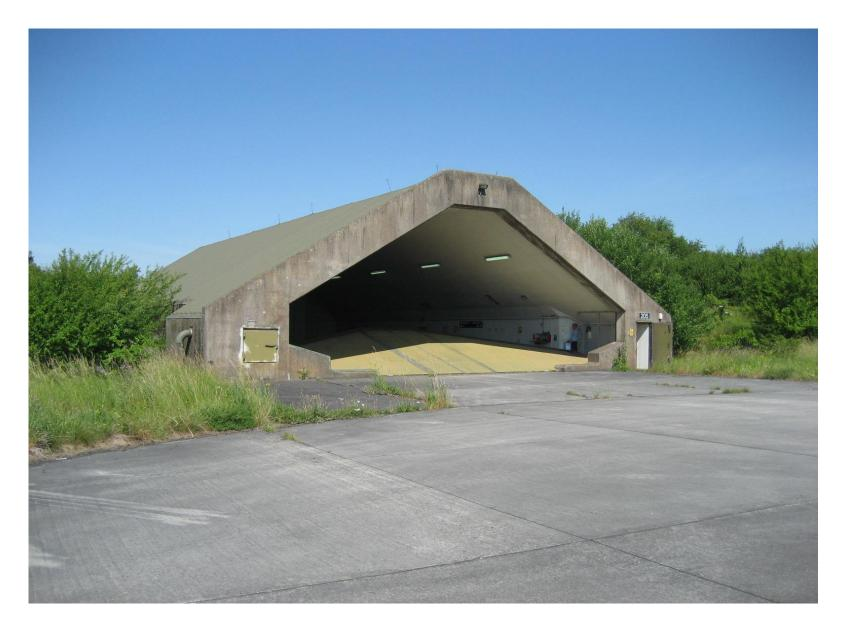
The roof is 50 cm solid concrete covered with plastic paint
